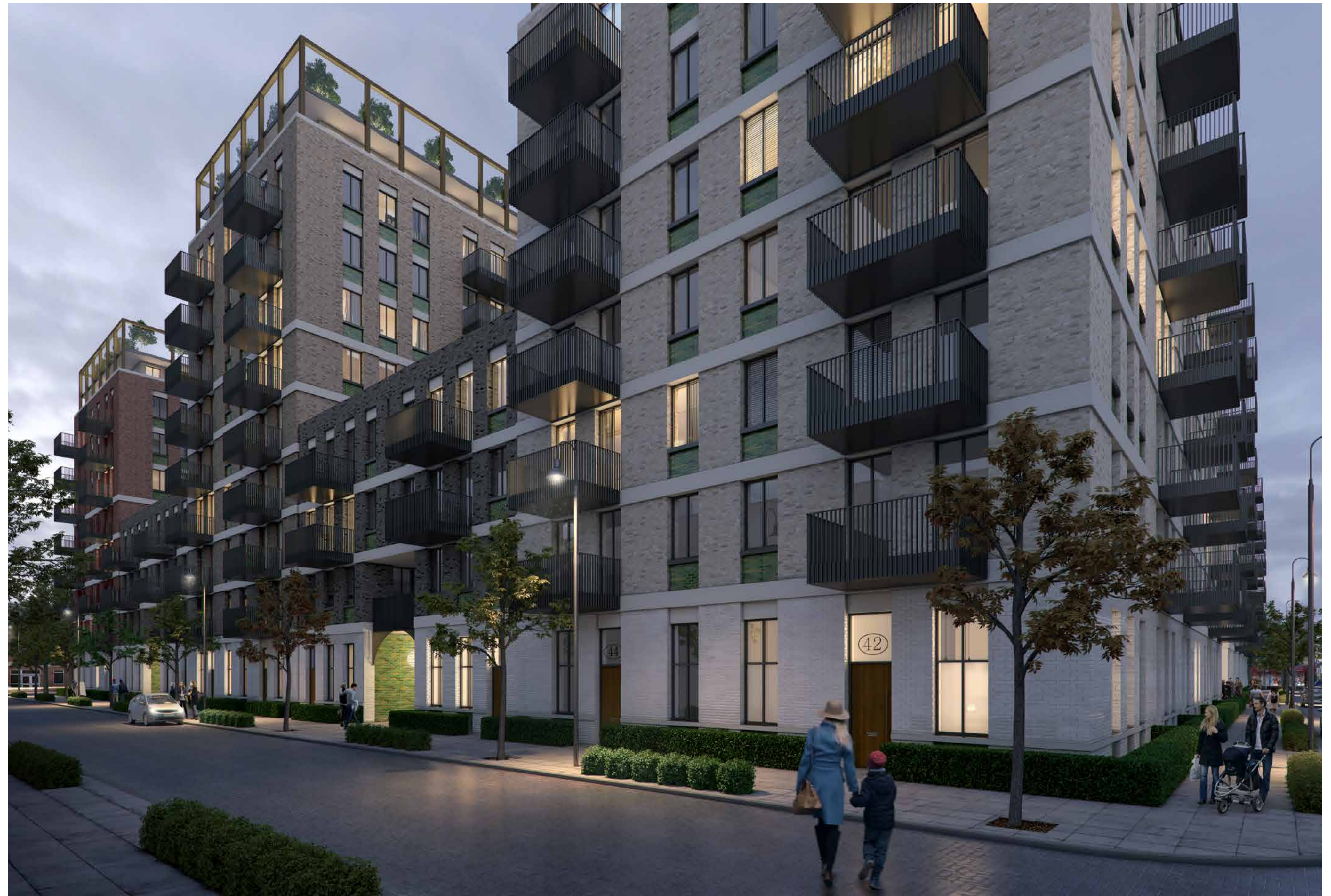
Indicative image of the view towards Morden Road
