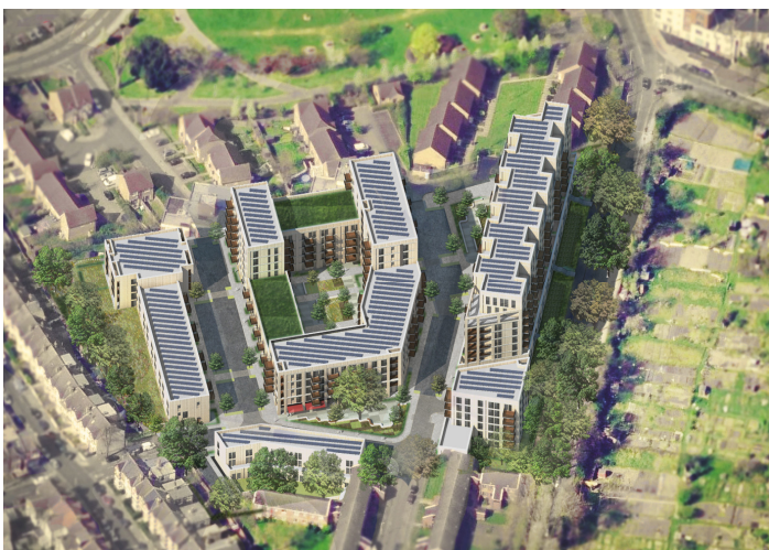
Aerial view of the new Sherwood Close
