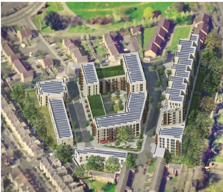
Aerial view of the new Sherwood Close
