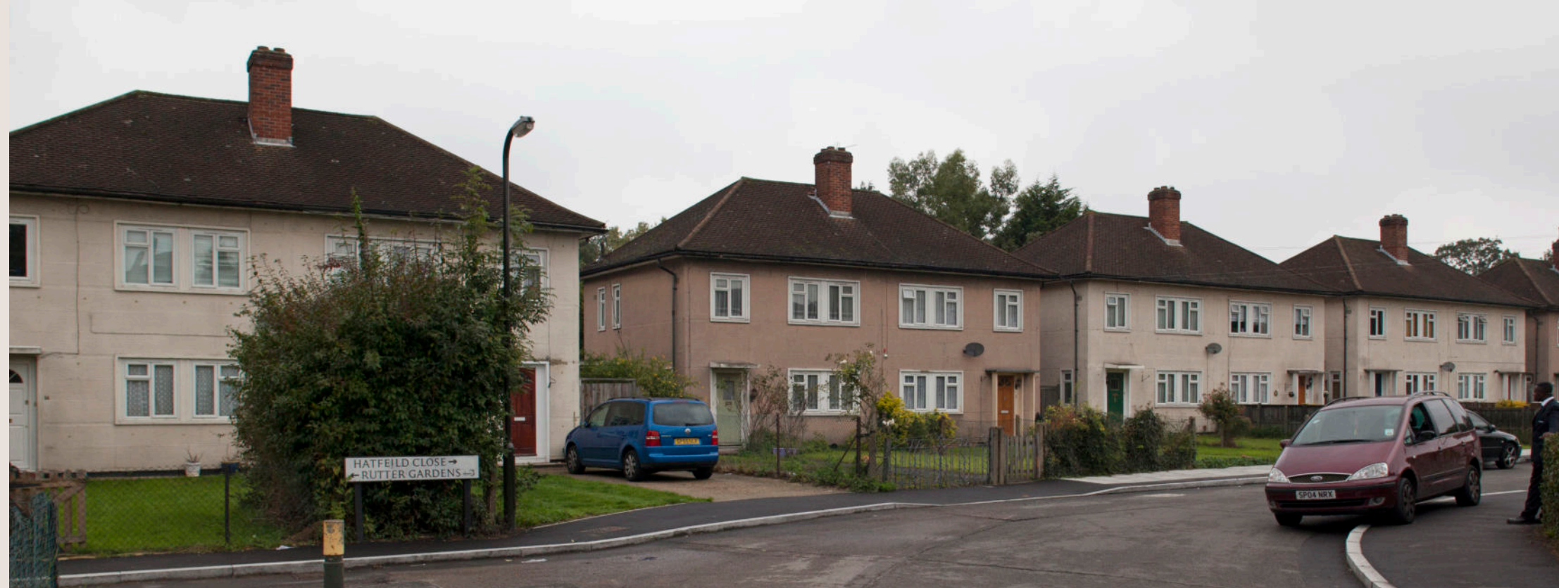
Existing vacant homes on Phase 3 site
