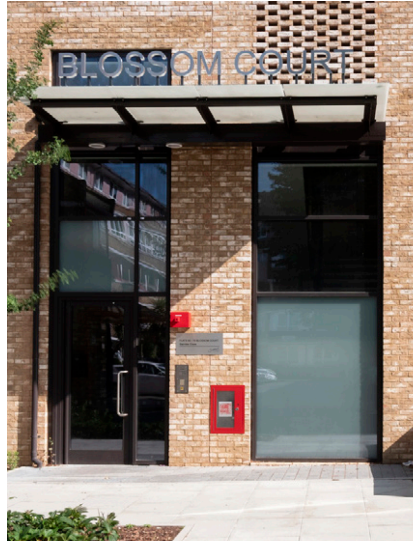
Typical flat block communal entrance
