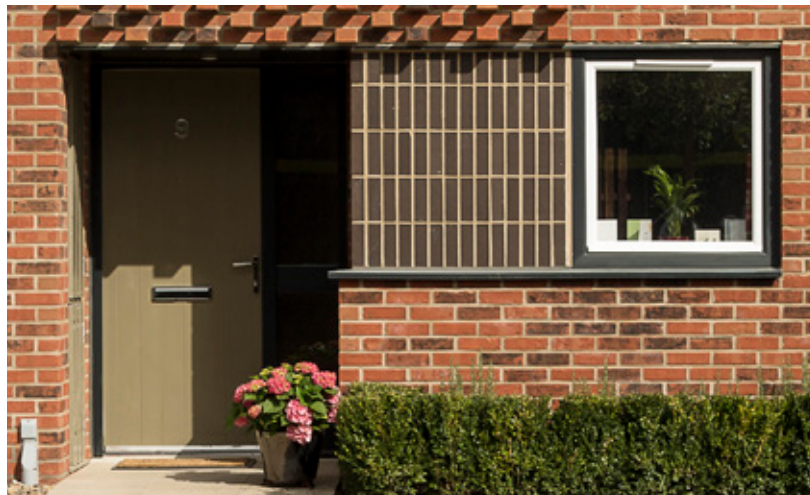
Typical recessed front door
