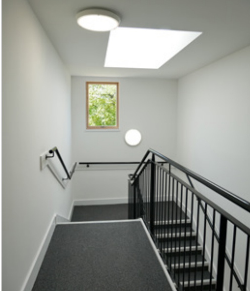
Typical communal stairwell
