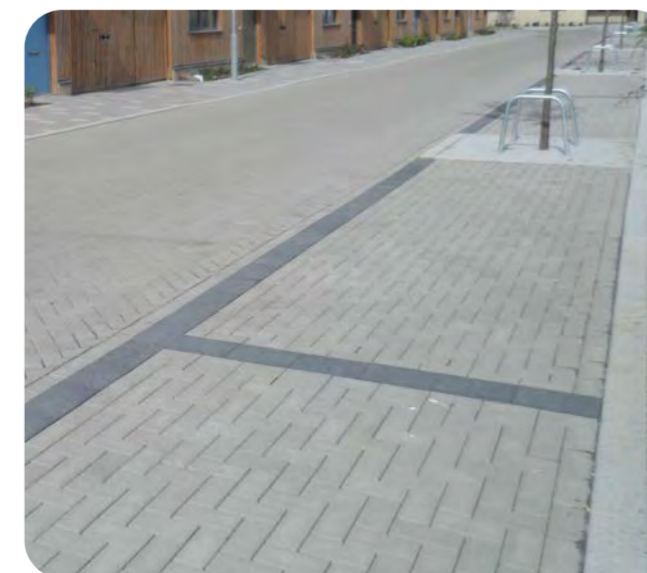
Belvedere - Block paving parking spaces
