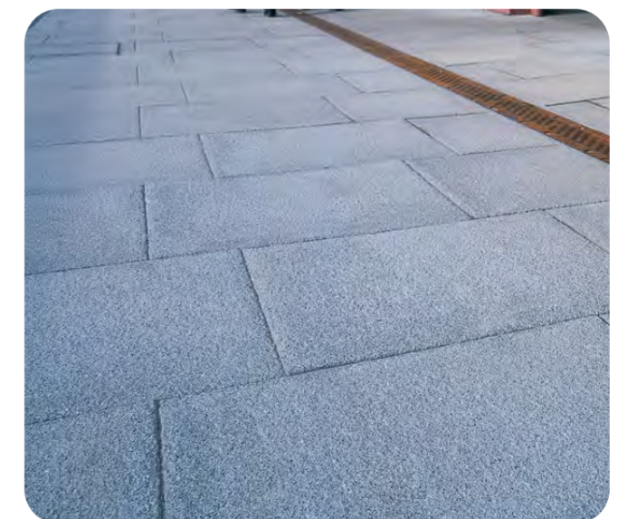
Belvedere - Slab paving pavements
