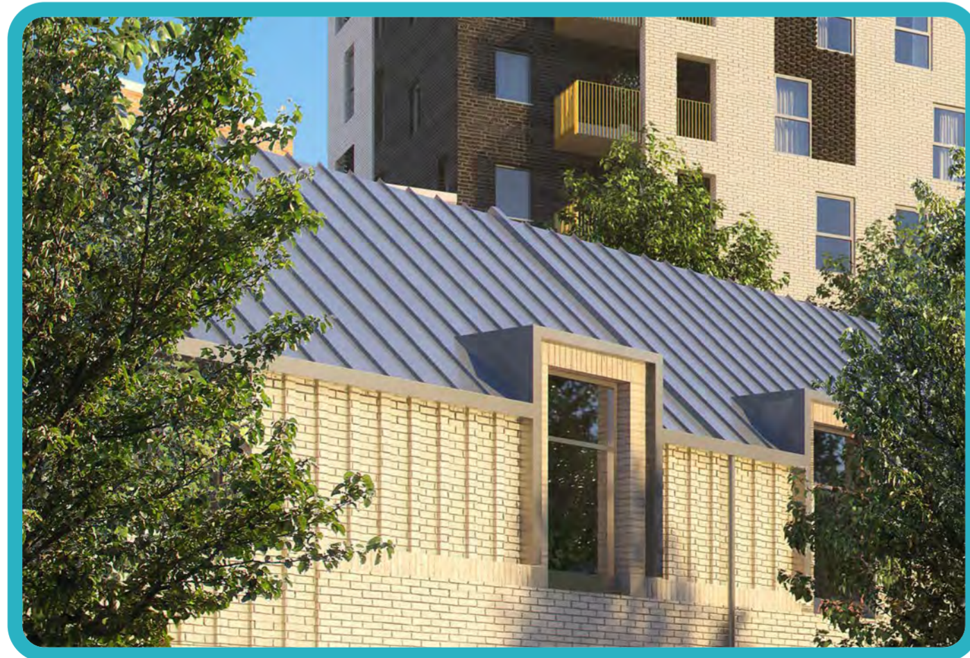
Link Street Roofs
